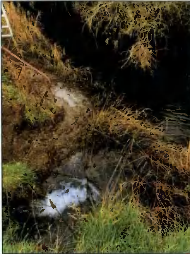
Plate 3-6. Outfall located at the Rye River
